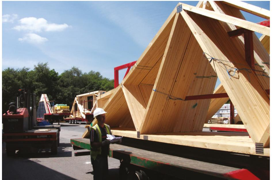
method is used, the units must not make direct contact with the ground or any vegetation. They must be arranged to avoid distortion, and securely restrained to prevent collapse.
